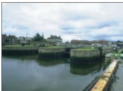
Recently restored Sea Locks
