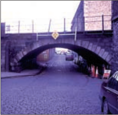
Restricted access under railway bridge
