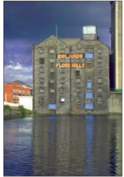
Bolands Flour Mills - a protected structure within Zone 7
