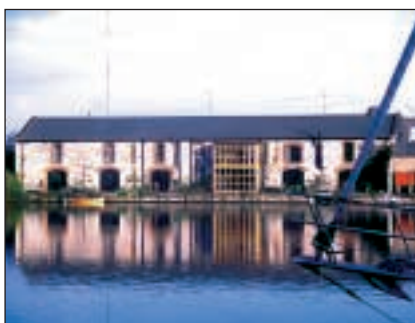
Protected structure on the quay of the outer basin
