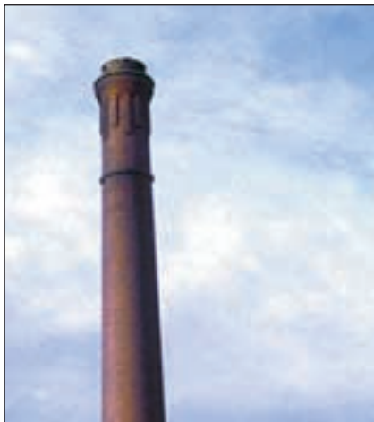
Chimney within Zone 2
