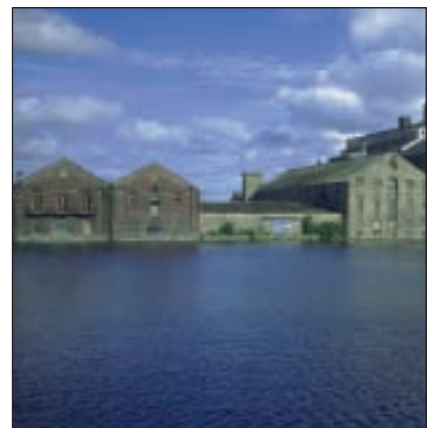
Warehouses within Zone 7
