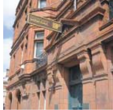
Former railway hotel
